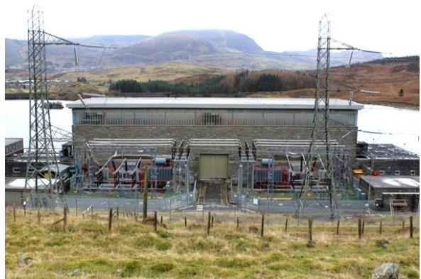
5: In the power station are the four large machines which can either pump water or generate electricity.
