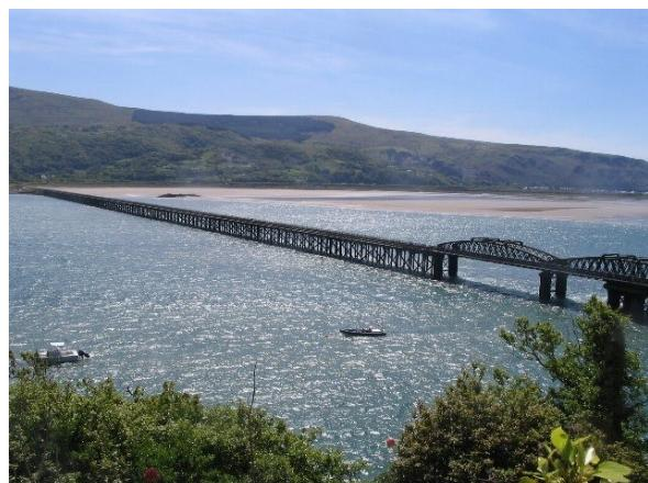
2: The main part of the viaduct is built of wood. Recent inspections have shown that both the wooden and iron sections of the viaduct require urgent repairs.
