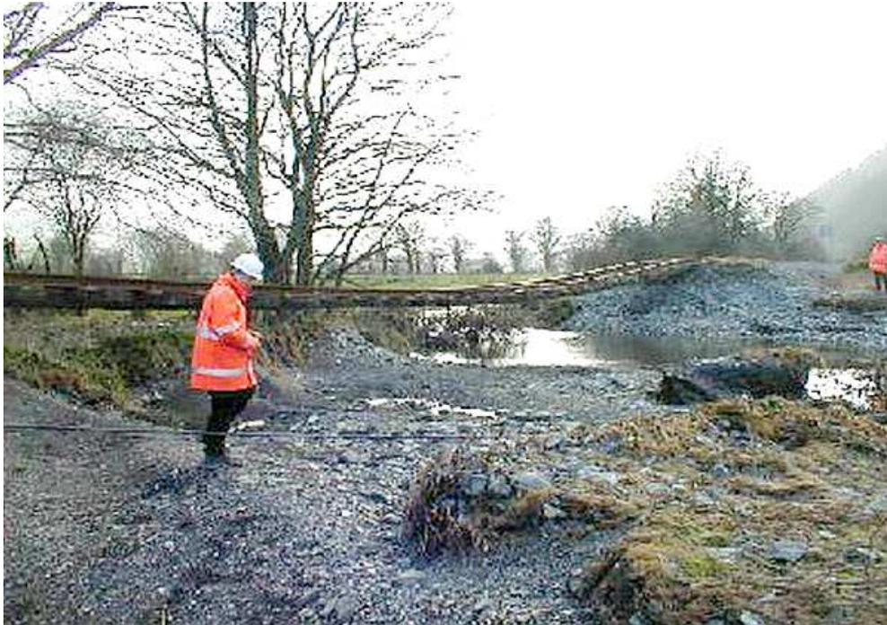
**Figure 2.48: Flood damage to the Conwy Valley railway line near Betws y Coed 4 February 2004.**
