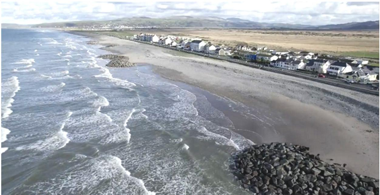
**Figure 54:** Boulder reefs providing coastal defences at Borth.
