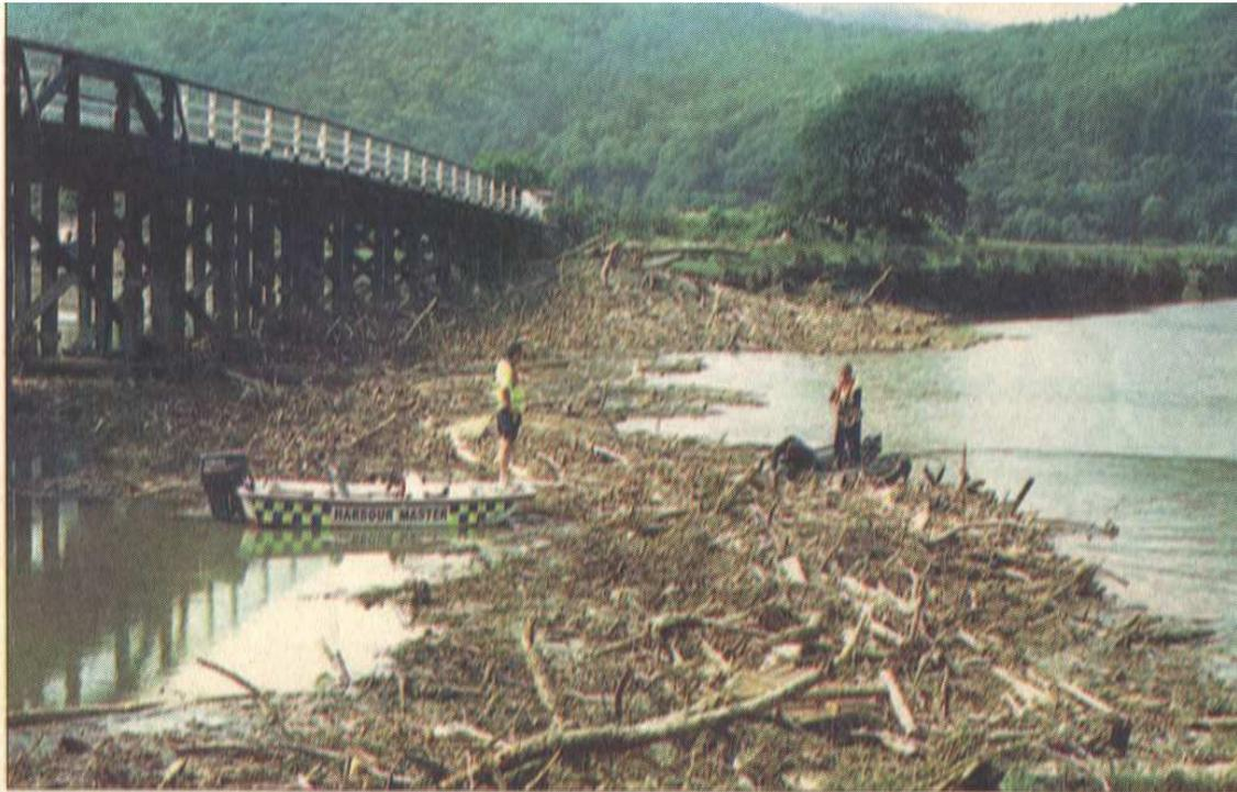
**Figure 3.256: Accumulation of forestry debris at Penmaenpool bridge from the July 2001 flood event.** Photograph: Cambrian News
